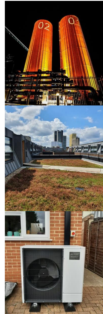
Images from top to bottom: The distinctive thermal stores at the ThamesWey energy centre Green roof at The Cornerstone refurbishment An air source heat pump installed for a resident through Green Jump Surrey
